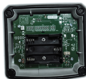
OMC-043-01 Power board (below solar panel)
